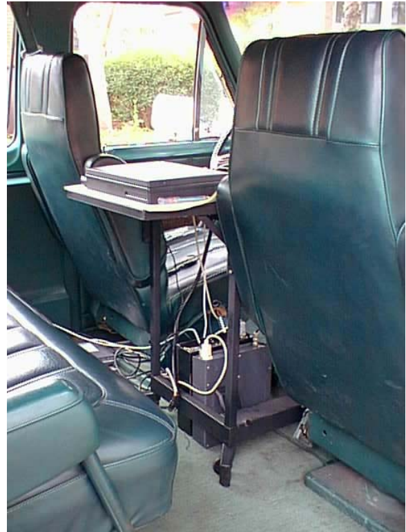
Figure 5. ISC Communications Equipment Installed in Van
